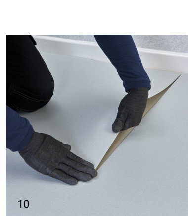
10 Once complete, place the floor covering into position ensuring a 'neat fit'.
