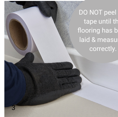
3 Apply the QuickLay double-sided tape around the perimeter of the room and at any doorways, set 2mm away from the edge of the room.
